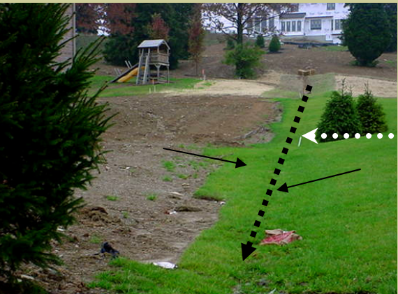
This swale was designed to allow rain runoff from adjoining property to flow toward the street, however, ...
