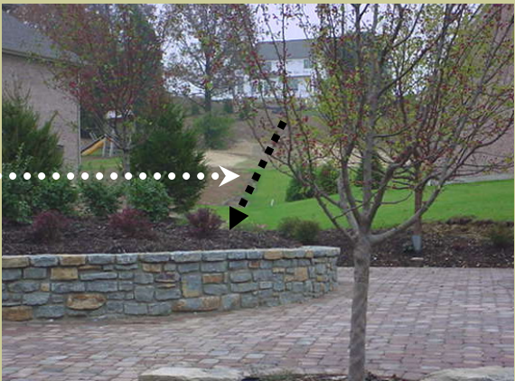
the installation of planters and paving above destroyed the natural drainage flow by blocking the swale.
