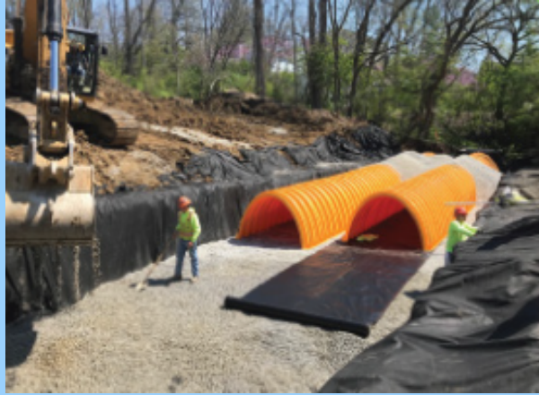
Installation of detention basin system at Clough Chase.
